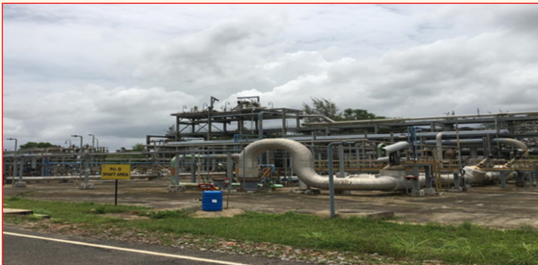
Shaft Area of Padur
