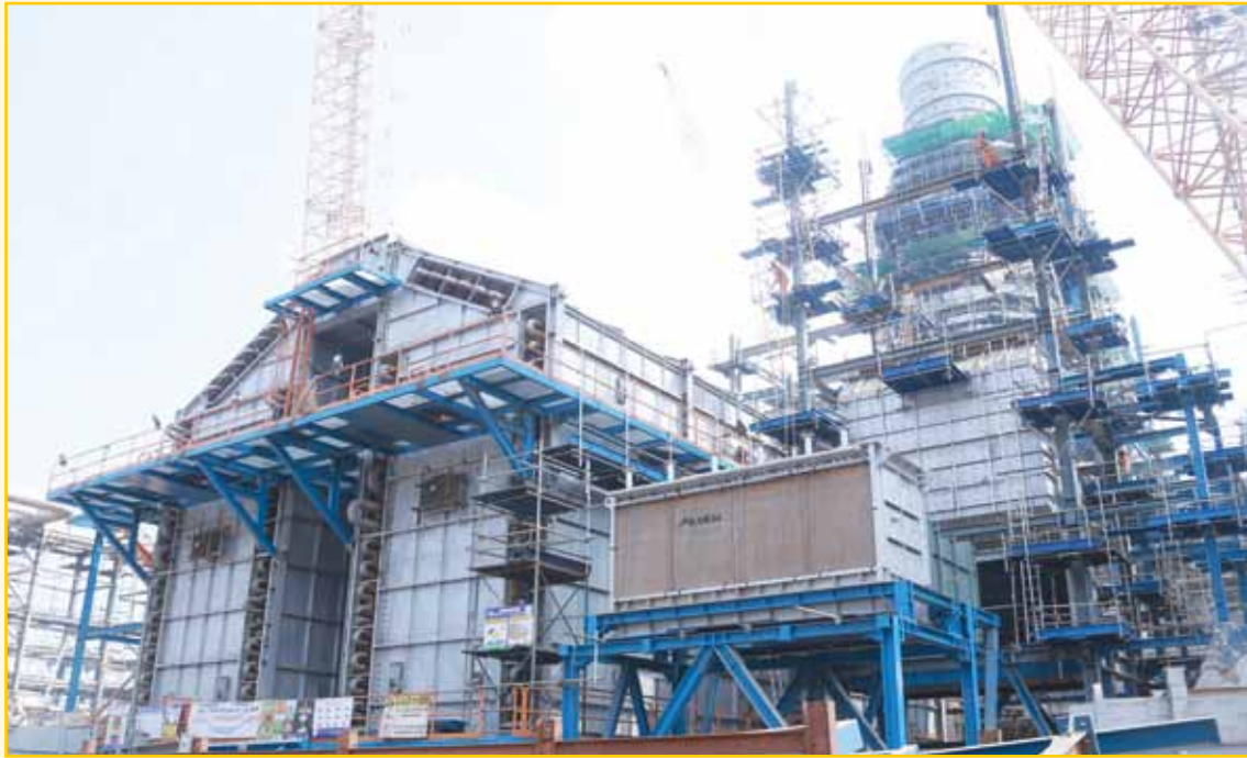
Visakh Refinery Modernization Project
